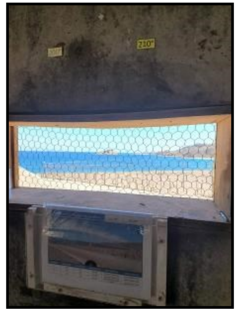
RS-3 Sangar looking to the South
